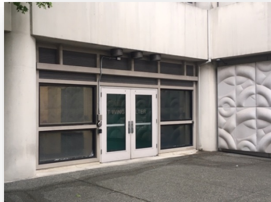
West Wing Shelter
